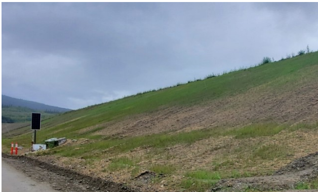
Hydroseeding on the Intermediate Dam in August 2023. Photo courtesy of CIRNAC.
