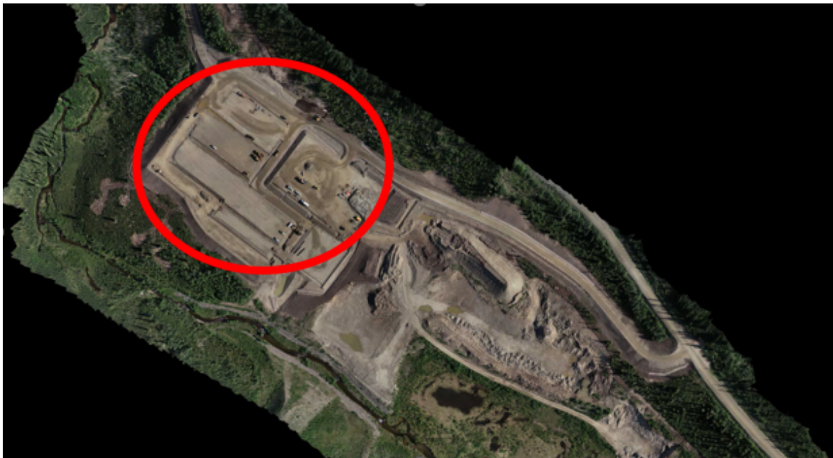
Aerial view of longer-term camp pad construction progress.
